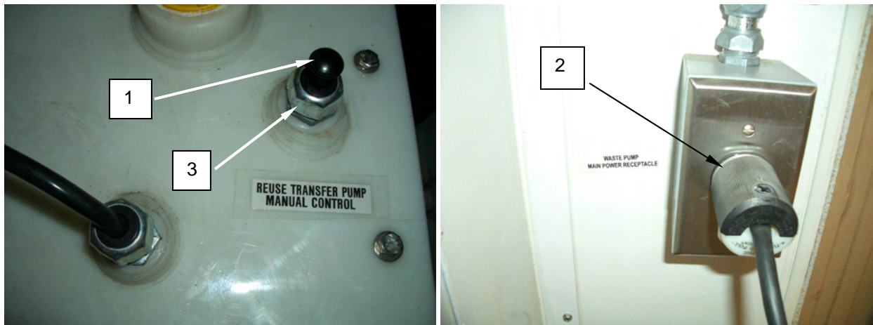
Figure 10. Loosening Watertight Tank Penetration and Pulling Wiring Through.
