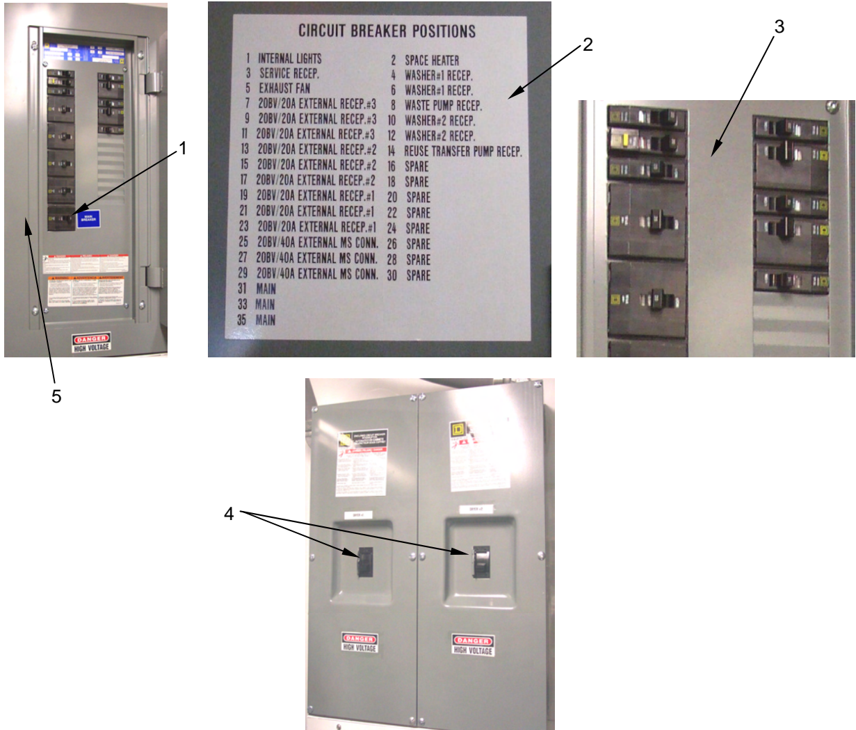
Figure 1. Test Circuit Breakers.
