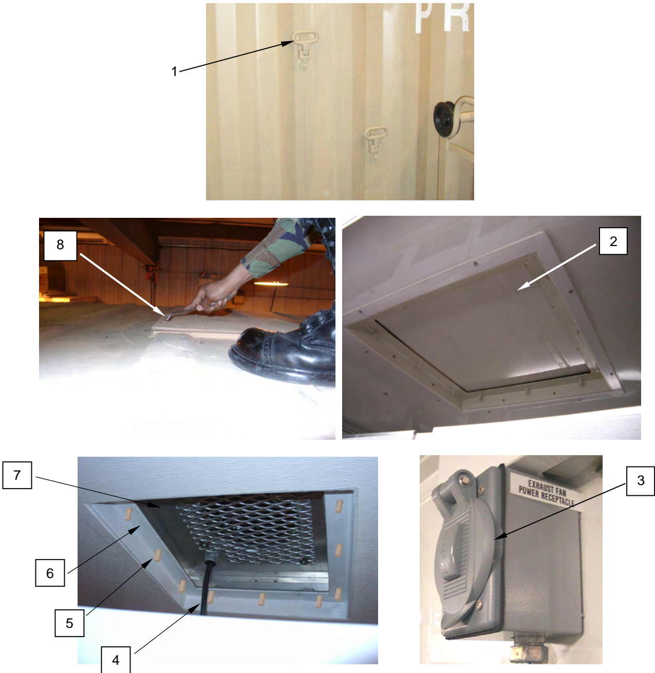
Figure 12. Installing the Exhaust Fan.
