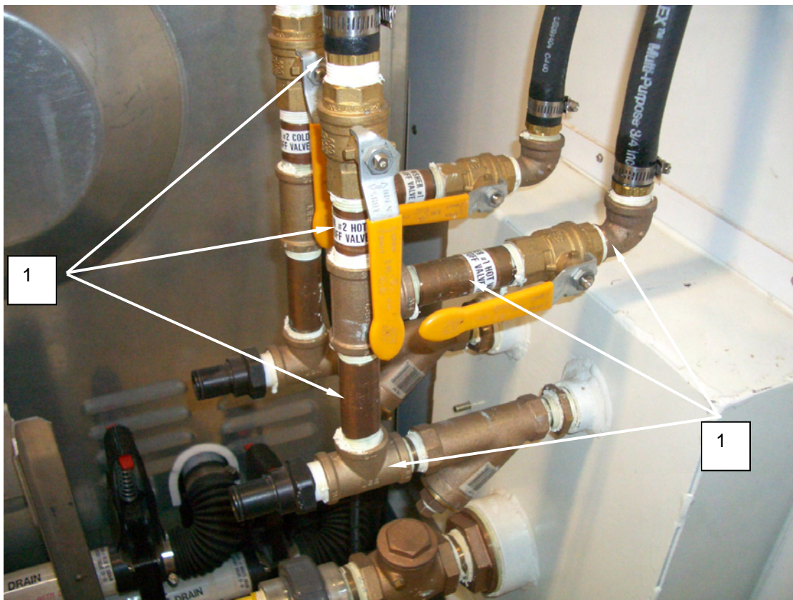
Figure 2. Replace Copper/Brass Pipe Fittings.
